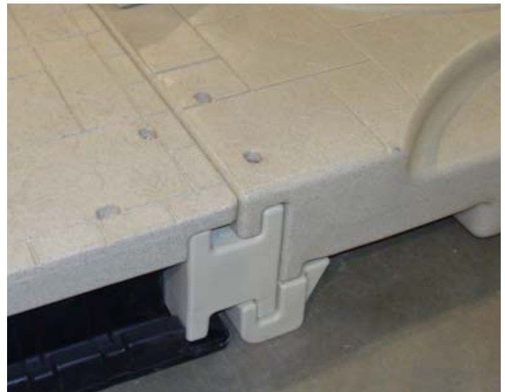
H-Beam in place
